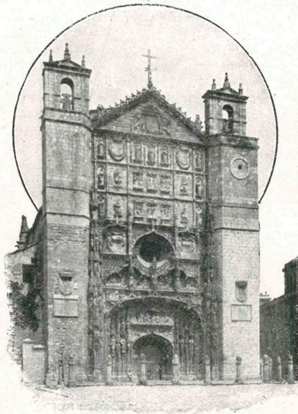
San Pablo (fachada principal)
